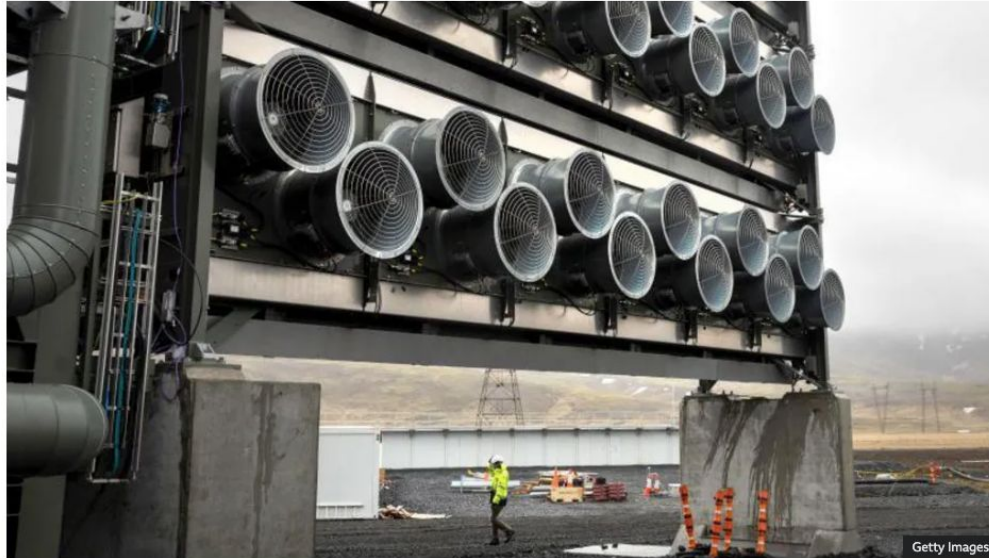
Climeworks' Icelandic plant captures CO2 direct from the atmosphere
